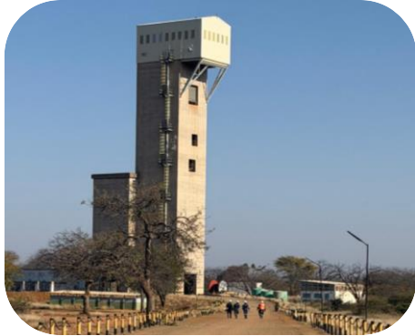
Selebi North (#4 Shaft) to 733 m level
