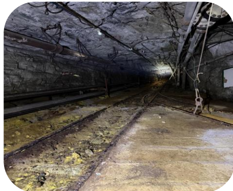
Cable belt conveyor to 850 level
