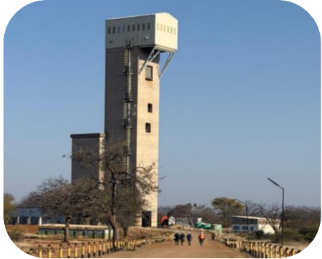
Selebi North (#4 Shaft) to 733 m level
