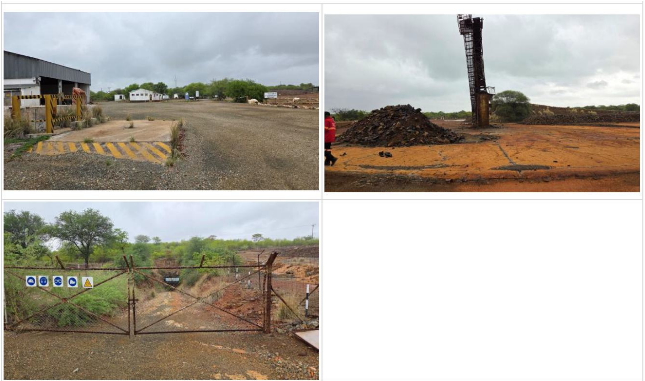
Figure 12-7 Historical infrastructure at Selkirk (workshop, conveyor and remains of massive sulphide dump, portal entrance)
