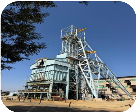
Selebi Main (#2 Shaft) 300 m level
