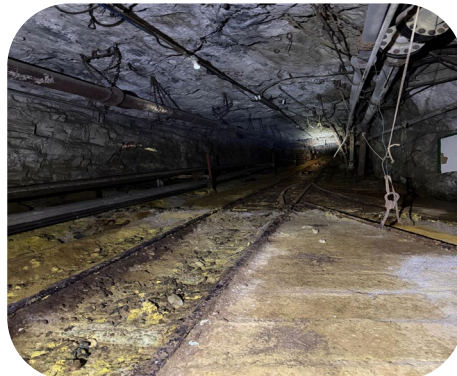
Cable belt conveyor to 850 level
