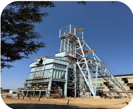
Selebi Main (#2 Shaft) 300 m level
