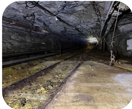
Cable belt conveyor to 850 level
