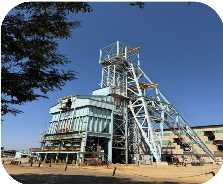
Selebi Main (#2 Shaft) 300 m level
