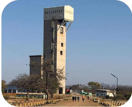
Selebi North (#4 Shaft) 745 m level
