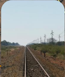
Grid Power and Rail
